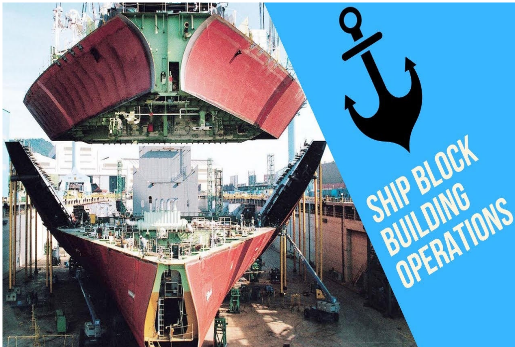
Figure 1: Typical block erection operation in a modern dry dock using heavy-lift cranes. Parallel block fabrication allows multiple units to be ready for erection when dock space becomes available.
