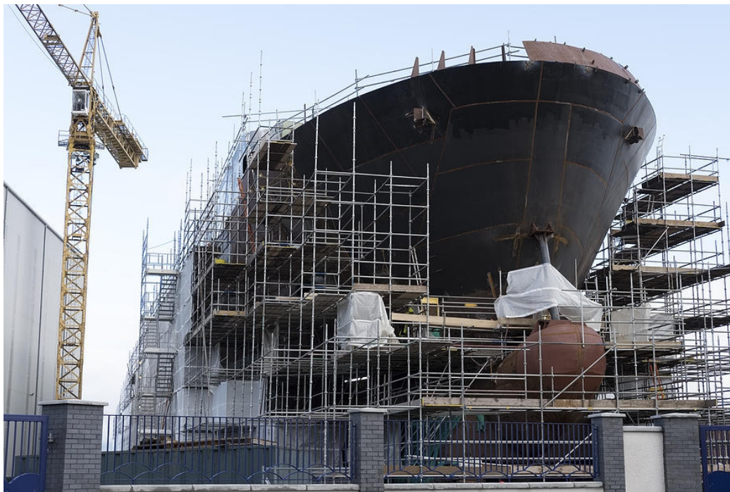
Figure 4: Dry dock environment showing block erection in progress. Careful sequencing and alignment control are essential to maintain structural fairness and schedule integrity.
